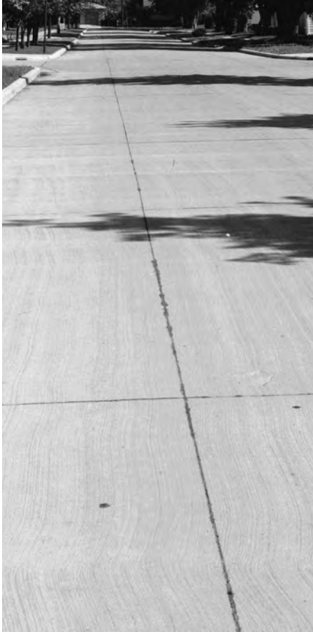
◀ New, well-sealed longitudinal joint.
