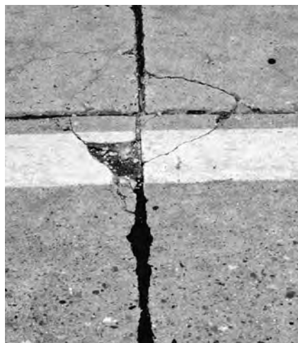
First signs of corner cracking.
