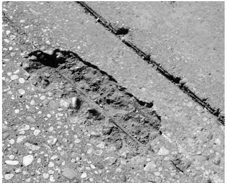
► Spalling over shallow reinforcing.
