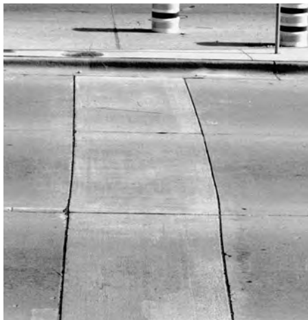
▲ Utility repair or full depth joint repair. Very good condition.
