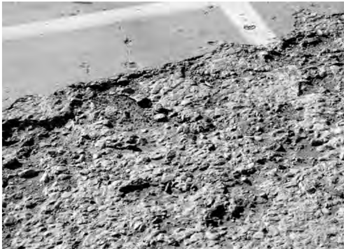
Reinforcing bar exposed. Shallow concrete cover caused large spall to develop around it. ▼
