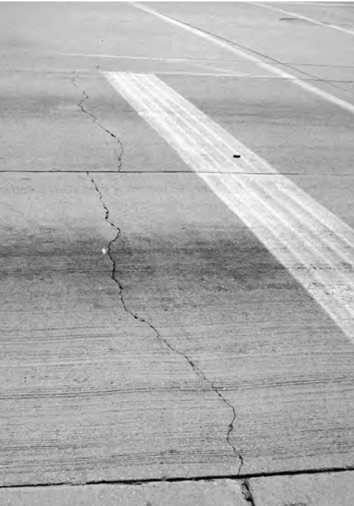
◀ Transverse crack. Tight, sound pavement.
