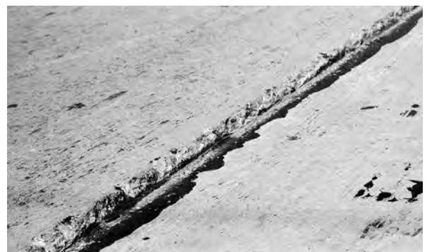
▲ Faulted longitudinal joint.
