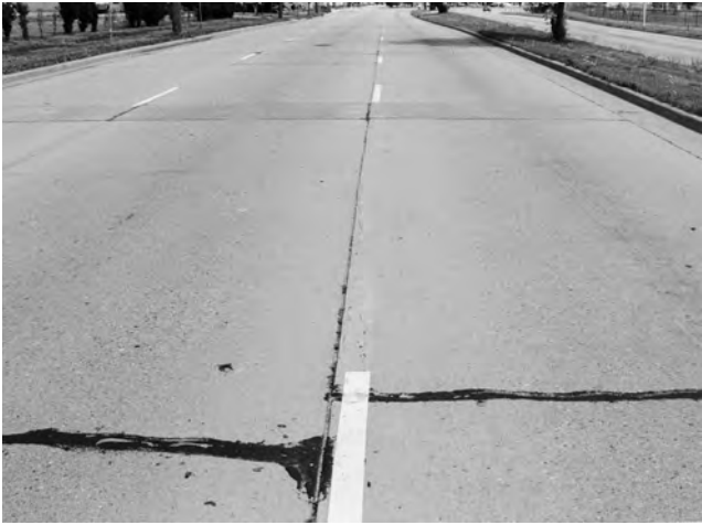
◀ Transverse crack. Tight, sound pavement.
