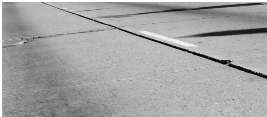
▲ Corner cracking developed into small hole; moderate spalling of transverse crack.
