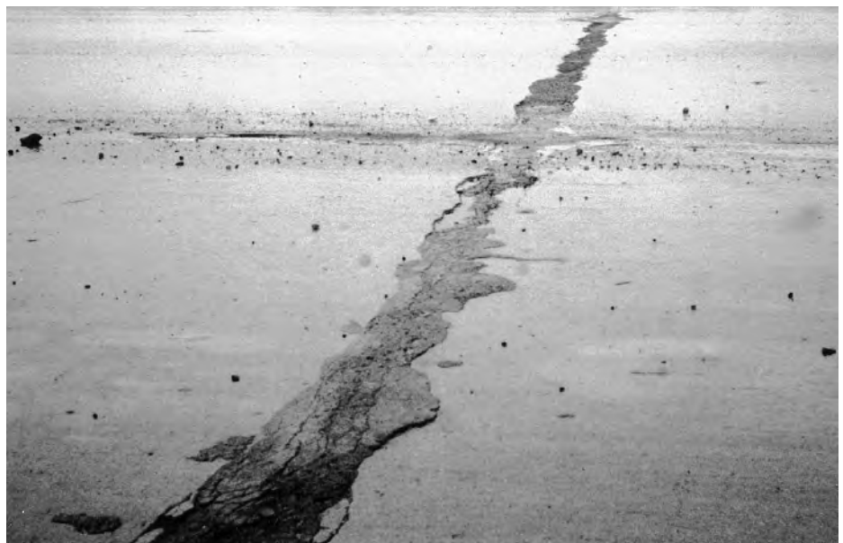
►► Cracks parallel to joint. Dark color next to transverse joint likely indicates D-cracking and additional deterioration. Full depth repair required.
