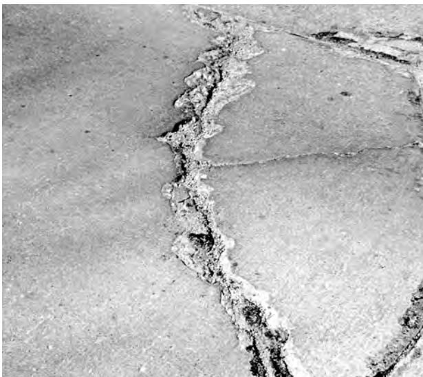
► Spalling over shallow reinforcing.
