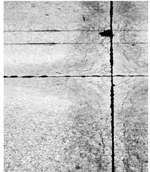
Surface discoloration near joints and cracks indicates D-cracking and severe slab deterioration.
