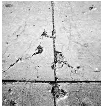
Corner cracking with broken concrete pieces.
