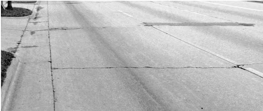
◀ All joints show some deterioration and spalling.
