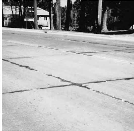
◀ All joints show some deterioration and spalling.
