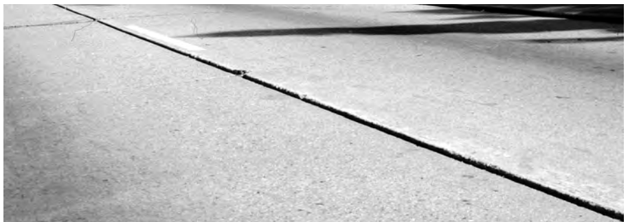
▲ Faulted longitudinal joint.
