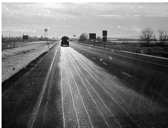
Typically anti-icing is a light application to dry pavement from streamer nozzles 12-18 hours before a predicted frost or snow event.
