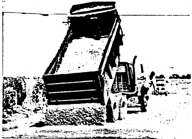
Figure 6. Under unusual conditions end dump trucks should back up while depositing gravel on geotextiles.
